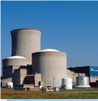
Power uprates and plant life extension
